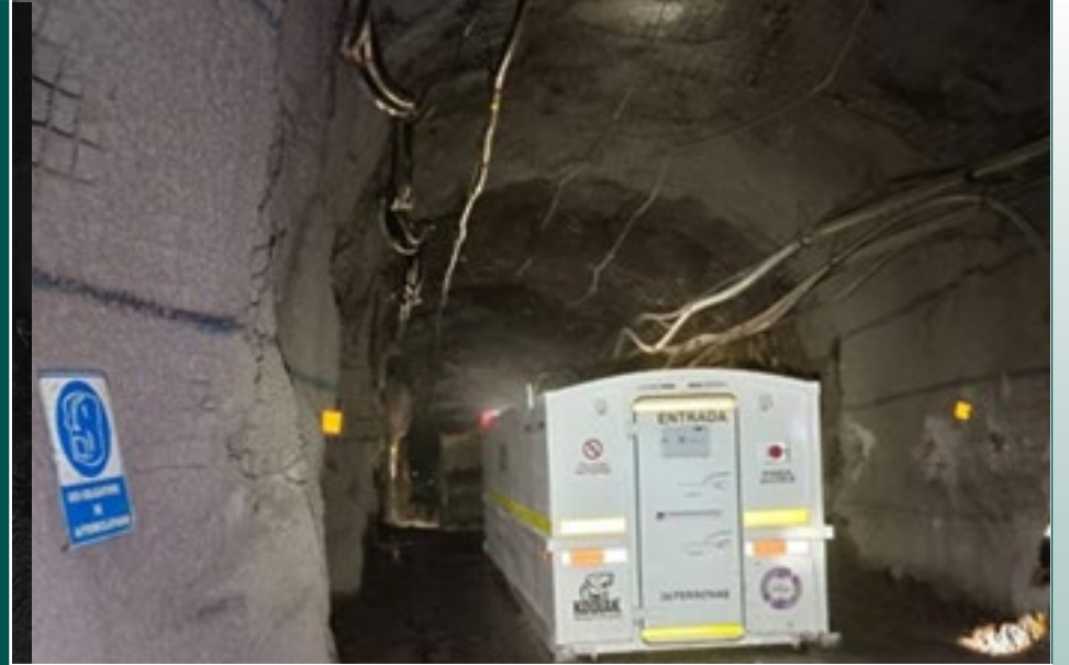
Installation of the rescue chambers
