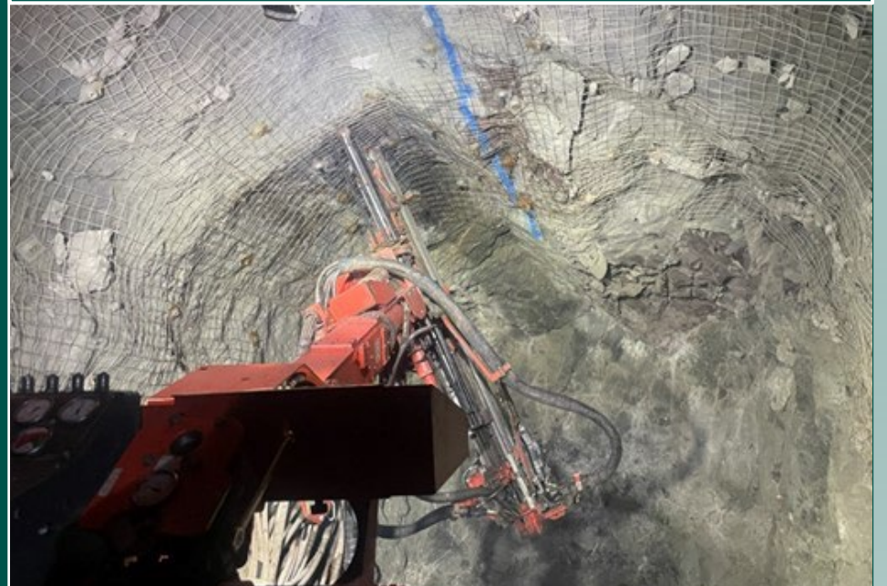
Bolter working in Portal 1
