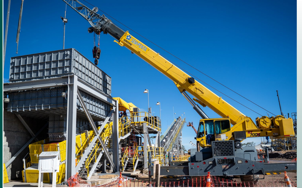
Feed chute installation for the primary crusher
