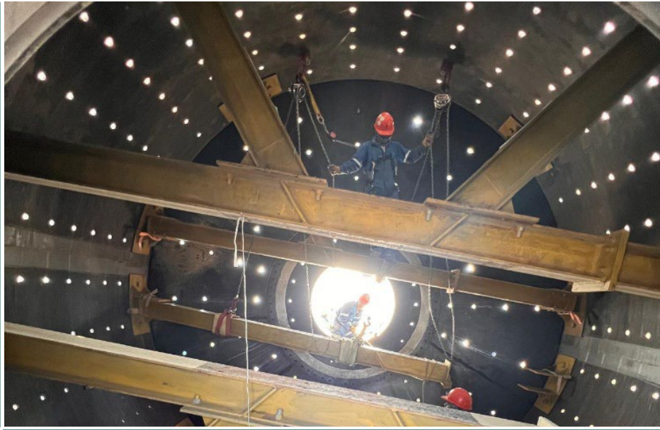
Inside the SAG mill prior to installing liners
