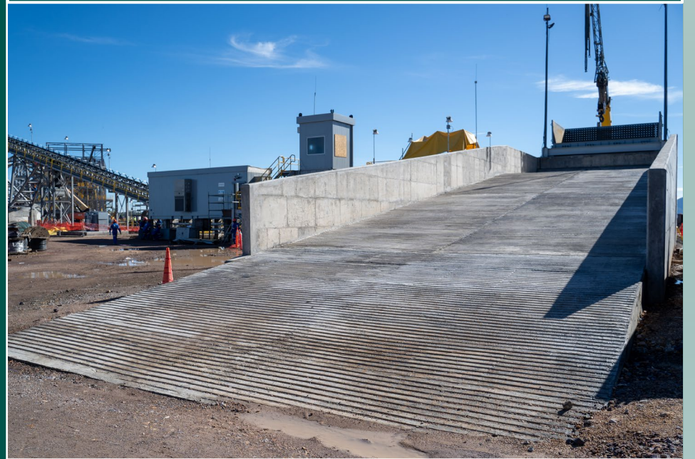
Loading ramp for primary crusher
