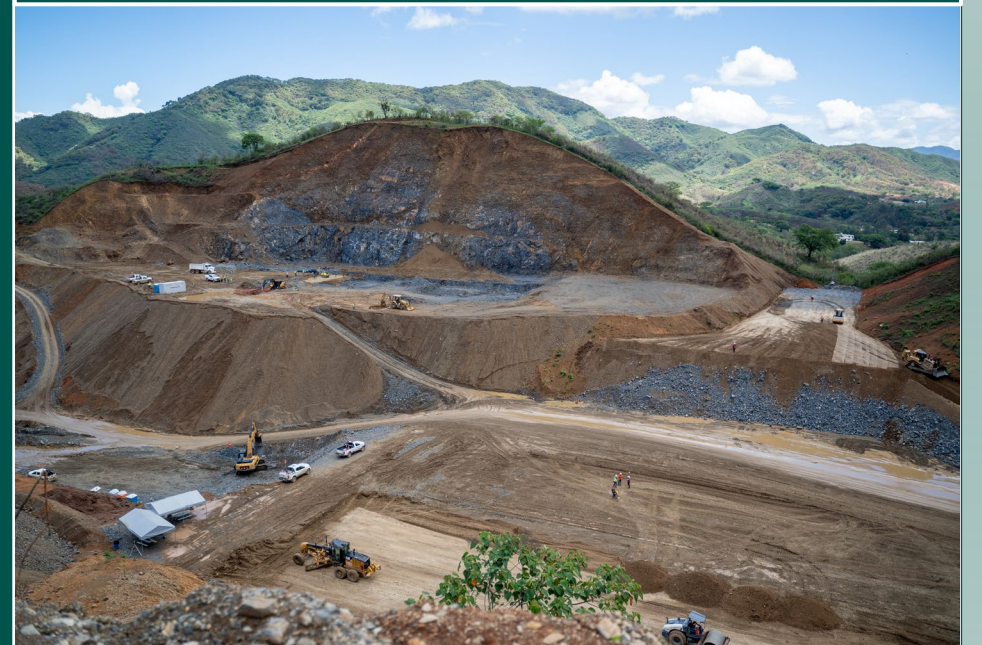
Above lower platform and filtered tailing embankment
