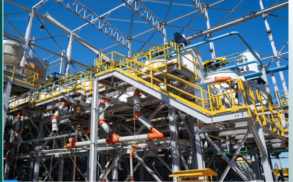
Piping installation well advanced in the flotation area
