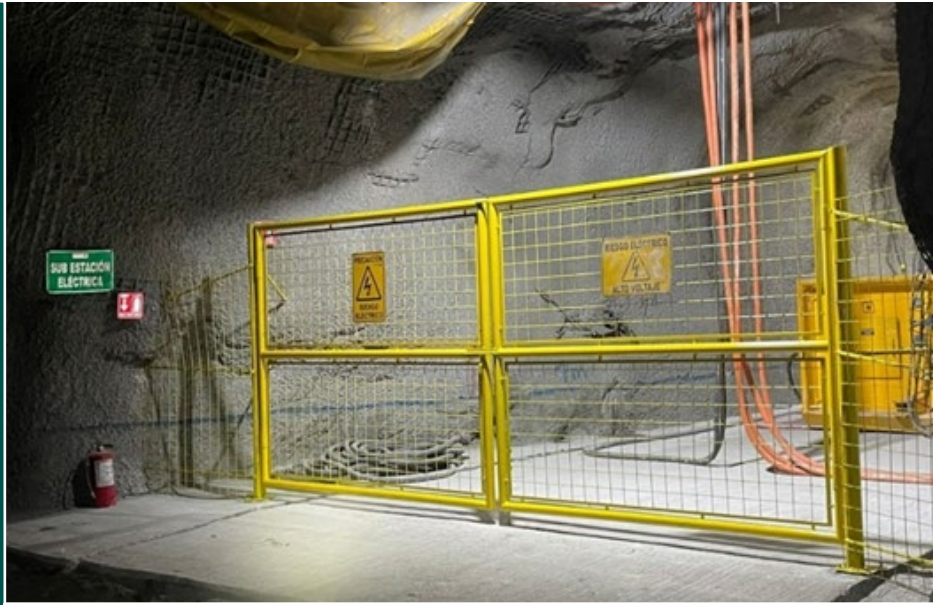
Installation of electrical substations
