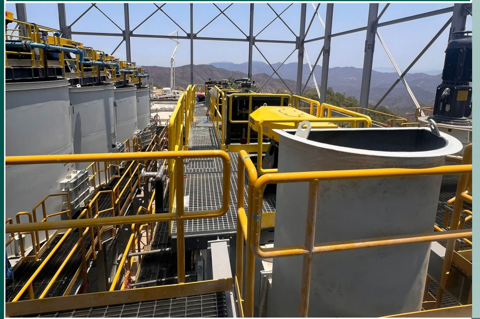
Flotation area well advanced from the upper deck area
