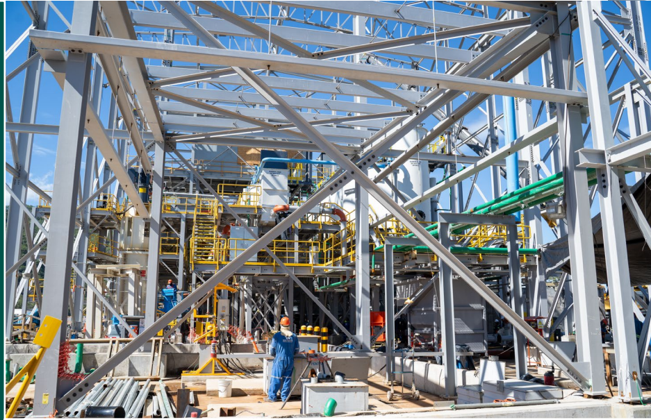
Installation electrical and mechanical equipment
