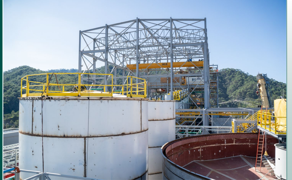
Raw and process water tanks welding over 90% complete
