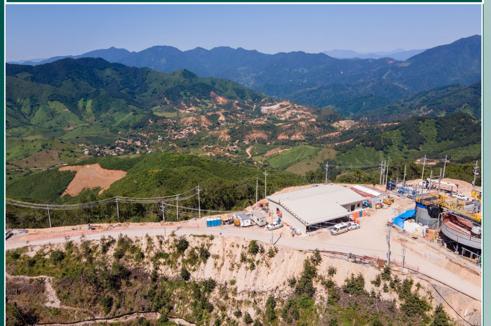
Assay and metallurgical lab, plant maintenance shop and thickener tank
