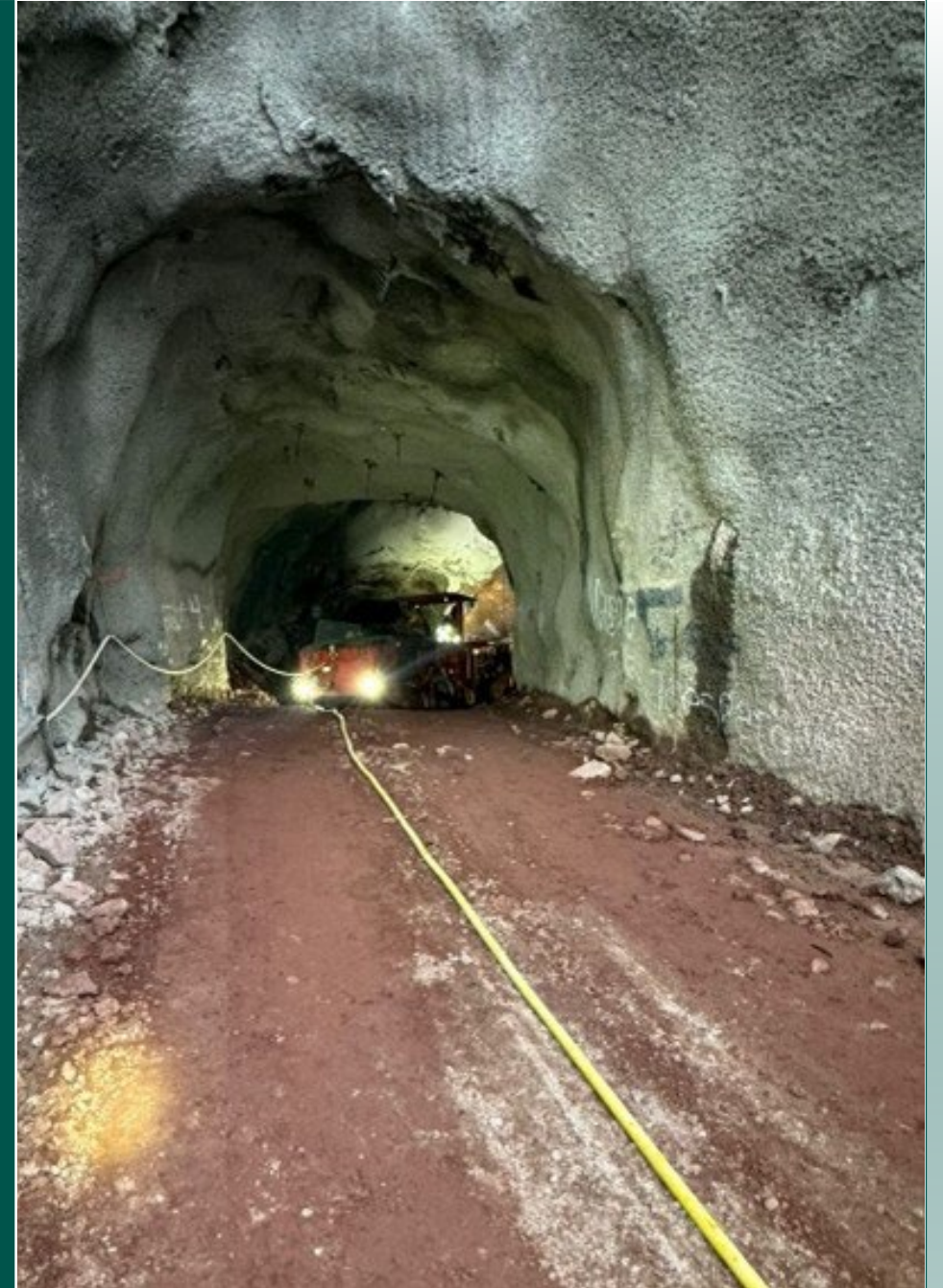
Portal 4 access work
