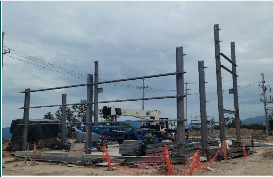
Plant maintenance building structural steel
