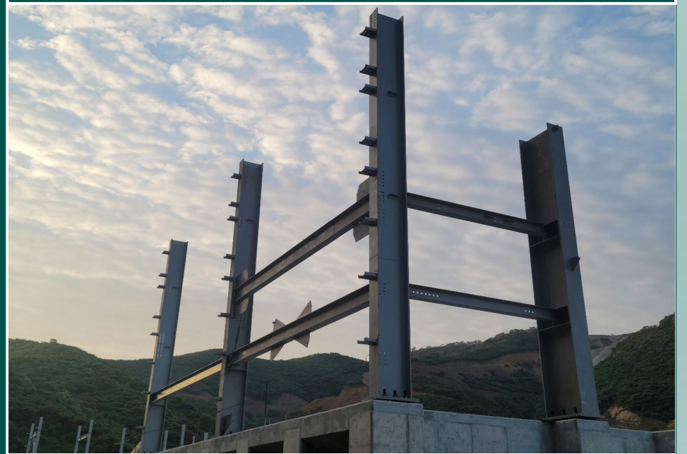
First tailing filter building structural steel
