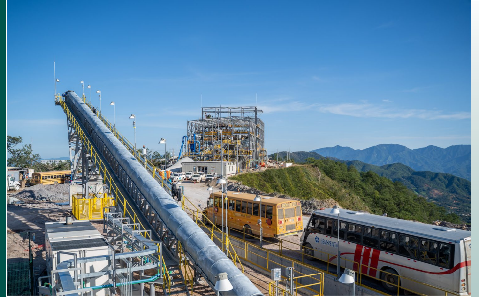
Conveyor – Primary crusher to coarse ore stockpile
