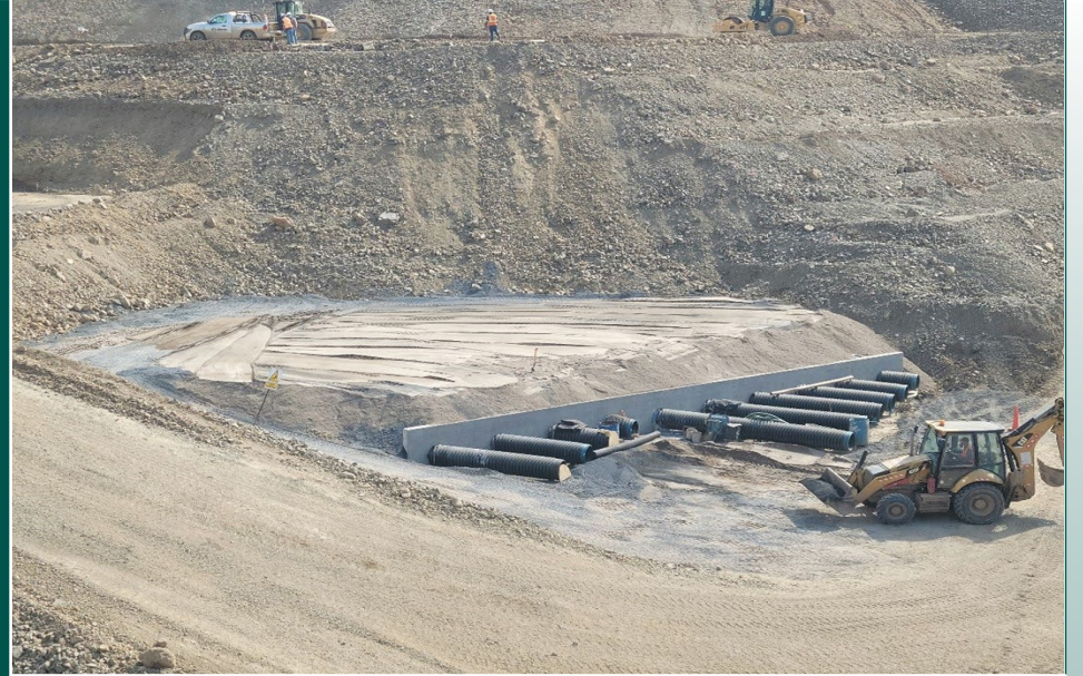
24-inch underdrain piping
