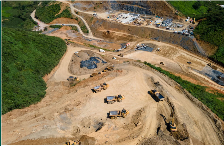
Above lower platform and filtered tailing storage facility
